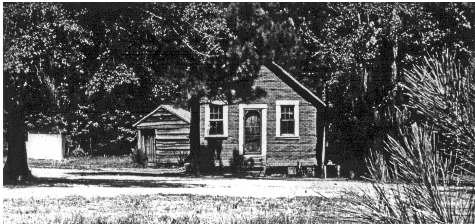
THIS ONE-ROOM NEGRO SCHOOLHOUSE, WHICH HELD 52 STUDENTS, WAS ABANDONED LAST SPRING
