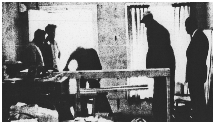
REMODELING THE OFFICE
