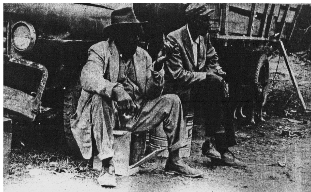
EVICTED PICKERS SAT AND WATCHED THE BULLDOZERS
