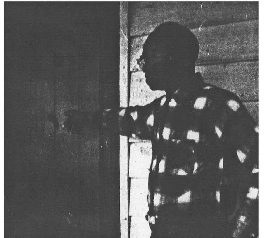
HOLES IN THE DOOR
