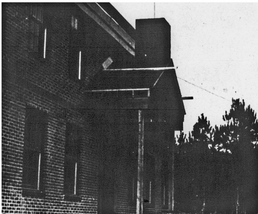
PICKWOOD ACADEMY BUILDING
