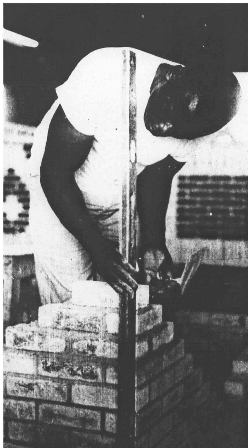
BUILDING A WALL
