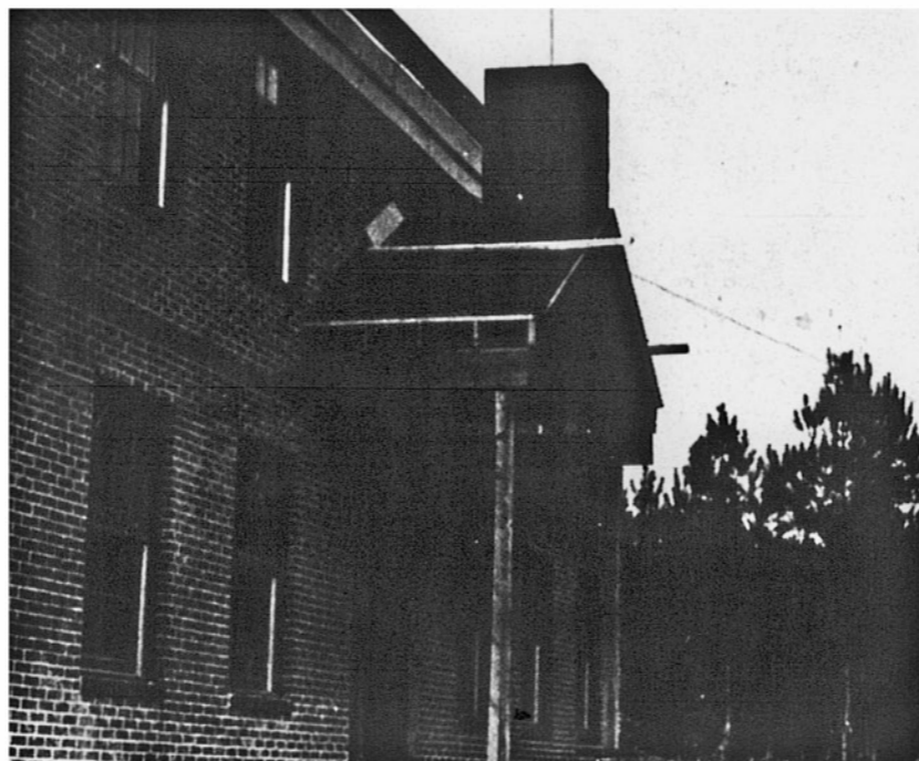
PICKWOOD ACADEMY BUILDING
