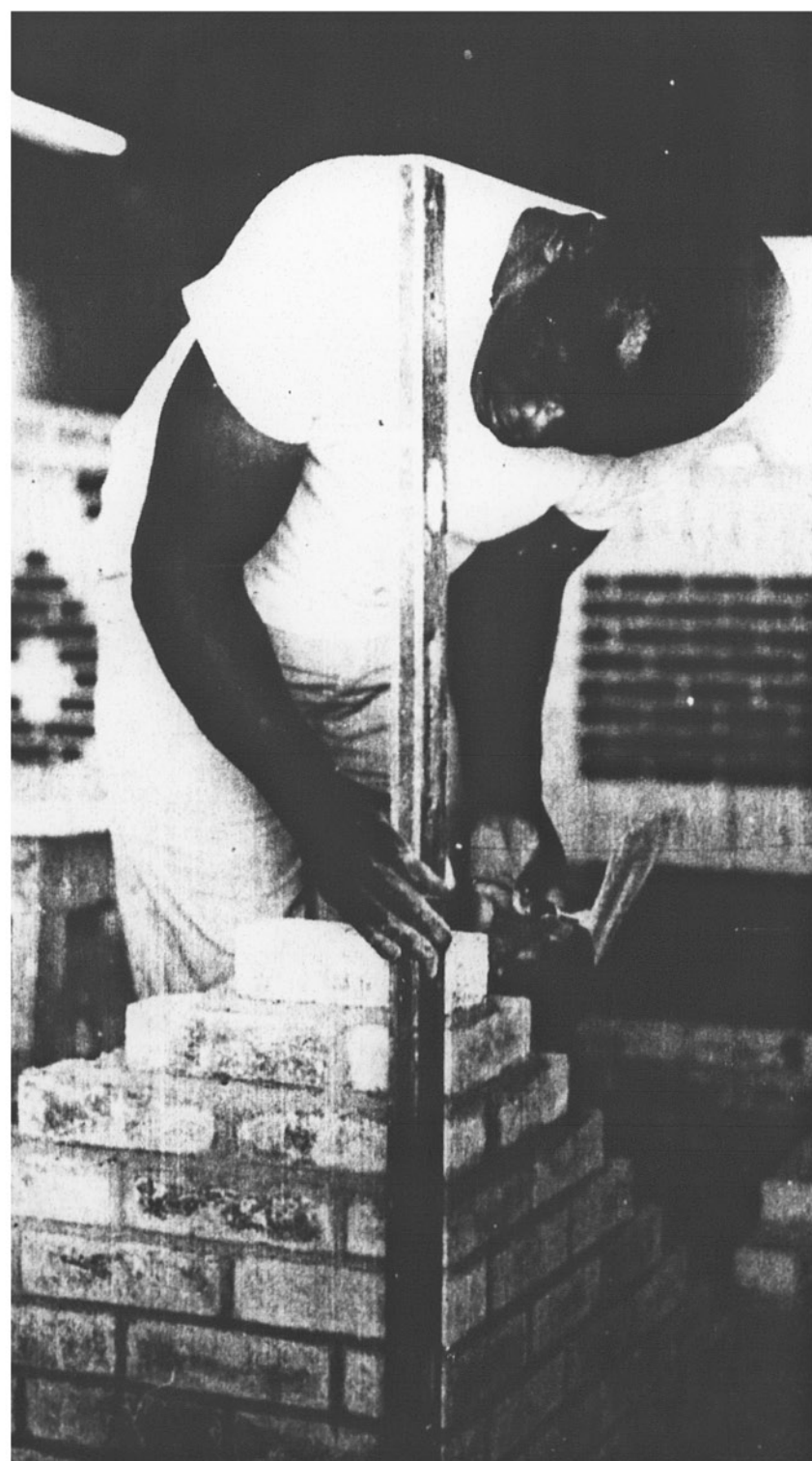
BUILDING A WALL
