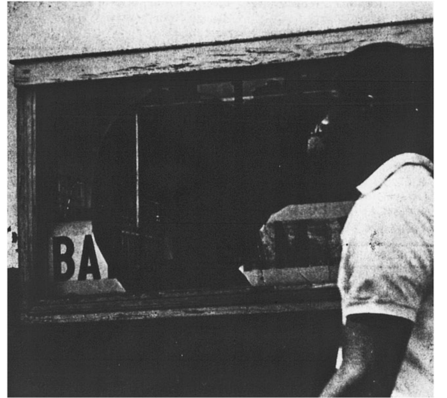
DAMAGE IN BIRMINGHAM
